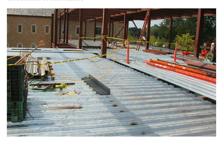
The five-year research program considered the seismic design of corrugated metal decks, with and without concrete topping, as a diaphragm system that is an integral part of the steel structure.
