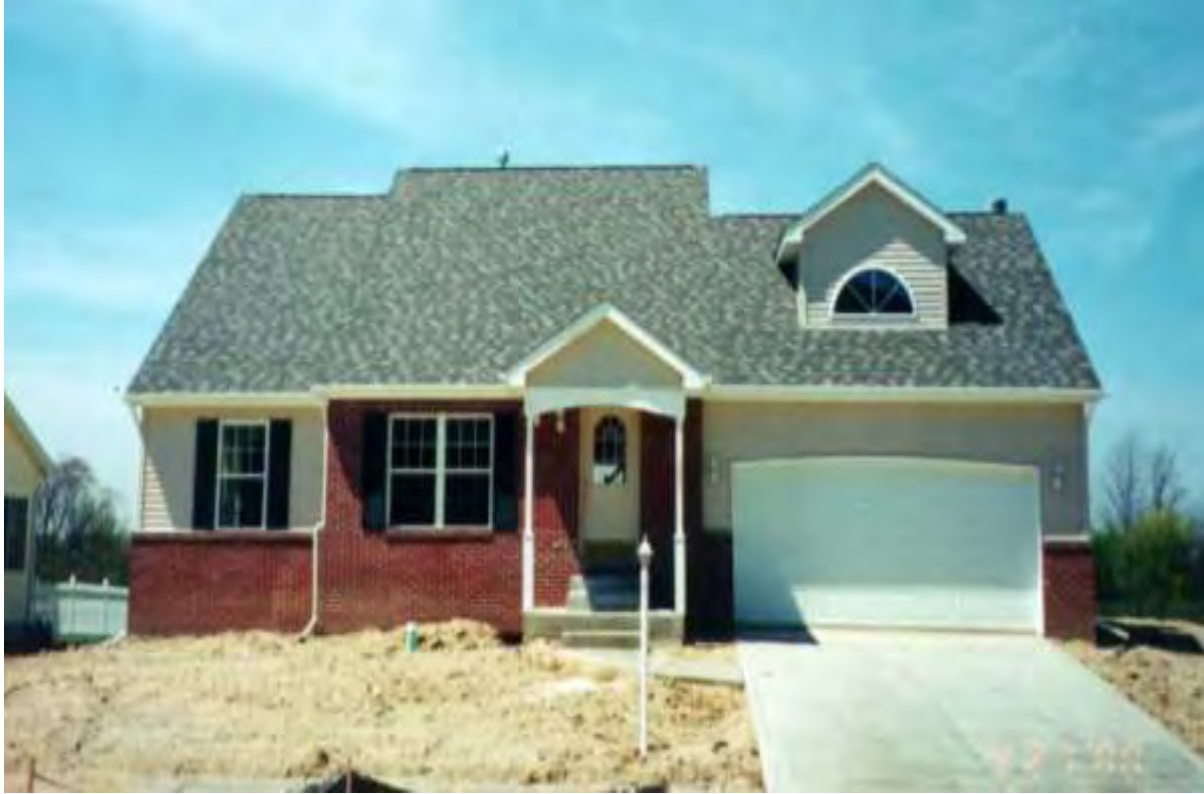
Figure 7: Wood Framed Demonstration House (NAHB Report)
