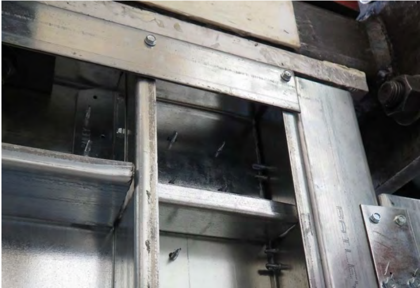
Figure 2.24 Final centre-sheathed configuration: stiffeners added in the corners
