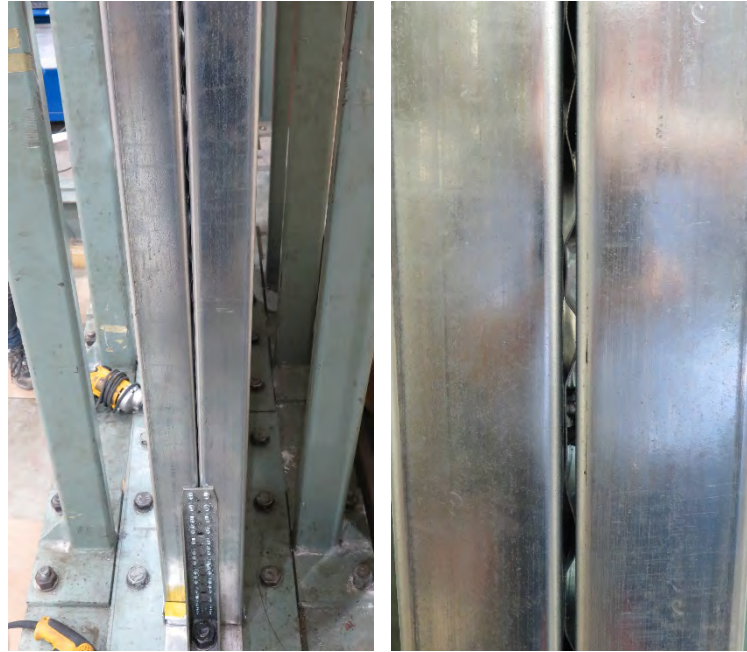
Figure 3.11: Centre-sheathed chord stud separation from sheathing shear buckling.
