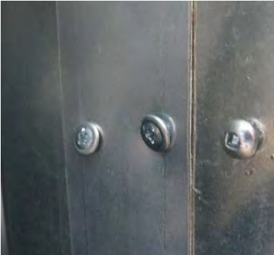
Figure 3.1: Tilting of built-up chord stud strap screws in a double-sheathed specimen.
