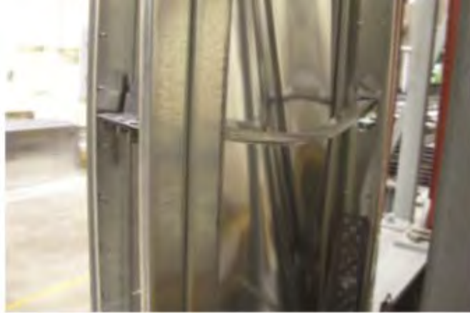
Figure 1.4: Buckling of bridging in CFS framed and sheathed shear wall (Balh (2010)).
