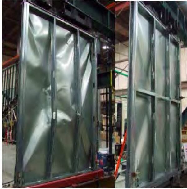
Figure 1.2 Failure mode of 6'x8' wall with (right) and without (left) special detailing (Yu & Chen, 2009)
