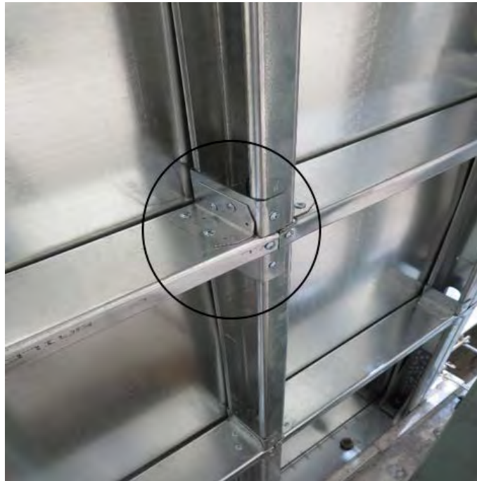
Figure 2.6 Blocking connection
