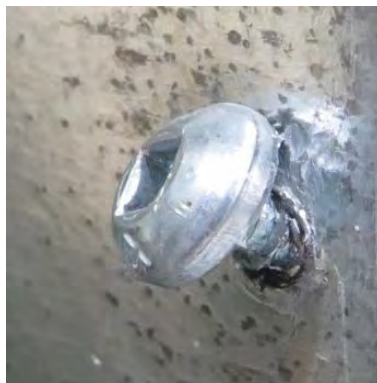
Figure 2.14 Sheathing screw tilting
