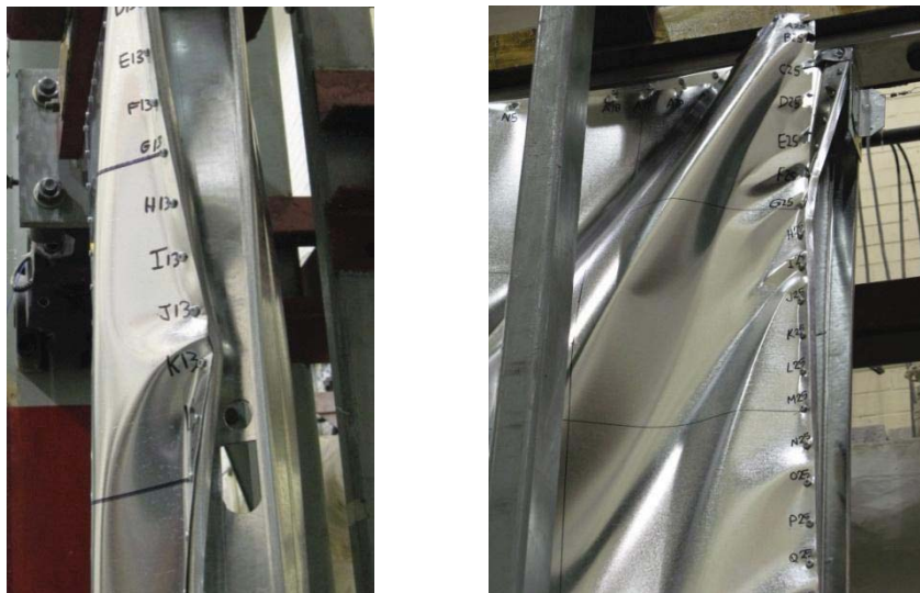
Figure 2.20 Twisting and Local Buckling of Chord Stud
