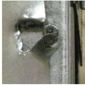
Figure 2.18 Screw Tear-out Failure
