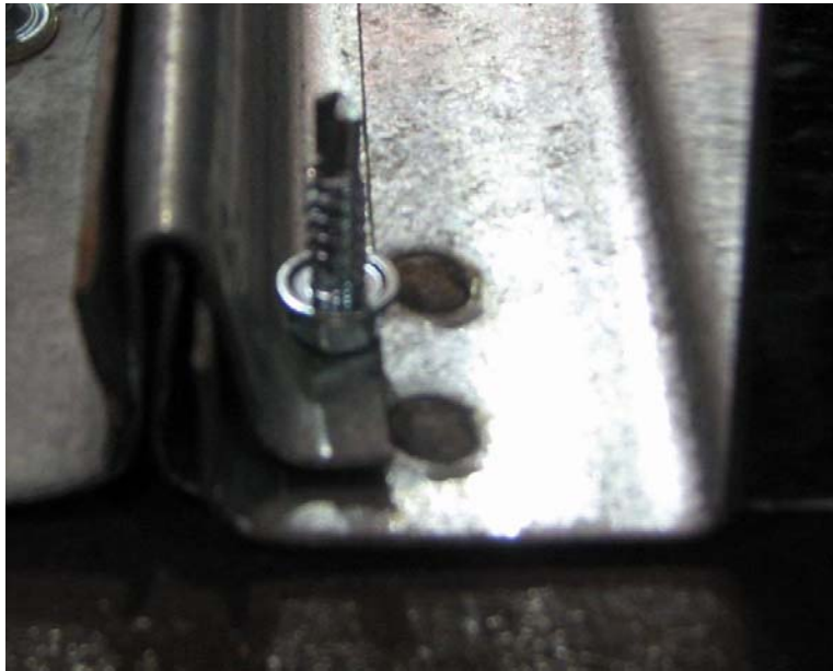
Figure 4-7: Side-lap Detail
