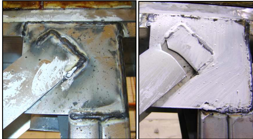
Figure 2.24: Medium wall strap connection prior to testing and after net section strap failure at 7.8% drift
