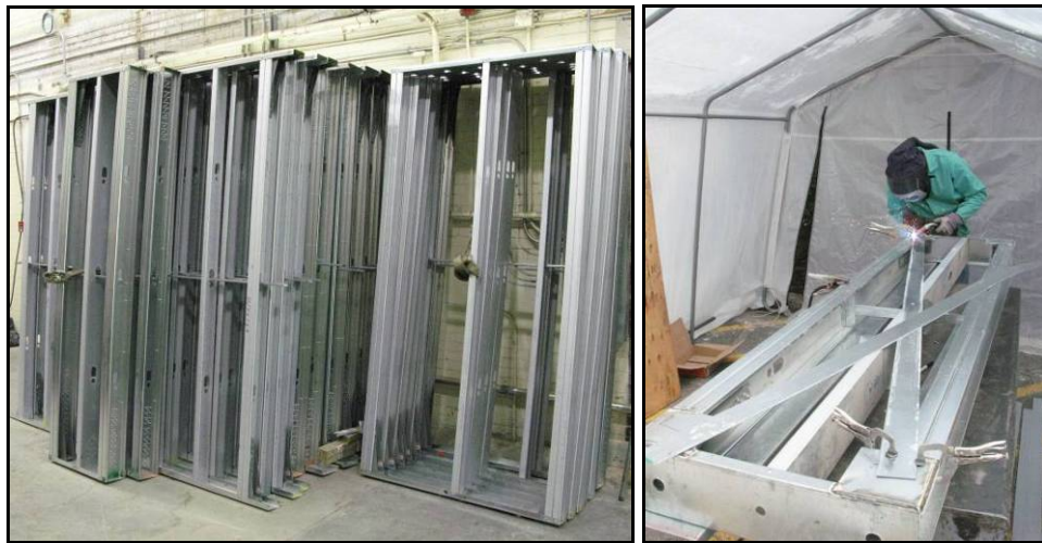
Figure 2.10: Assembled walls in laboratory; final welding of gusset plates and straps
