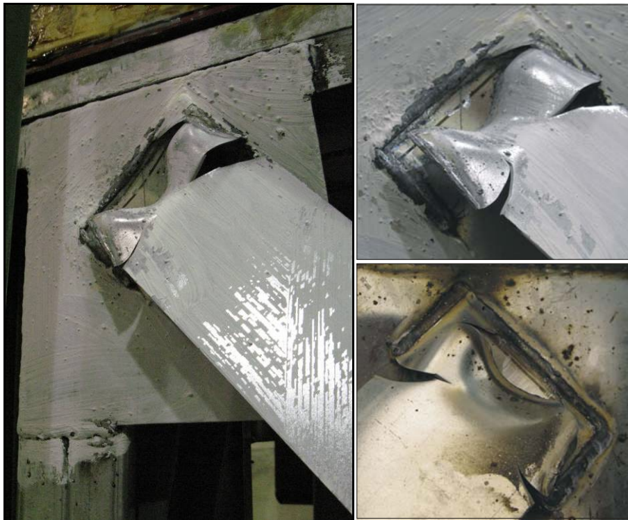
Figure 2.13: Connection failure of preliminary test 21A-M
