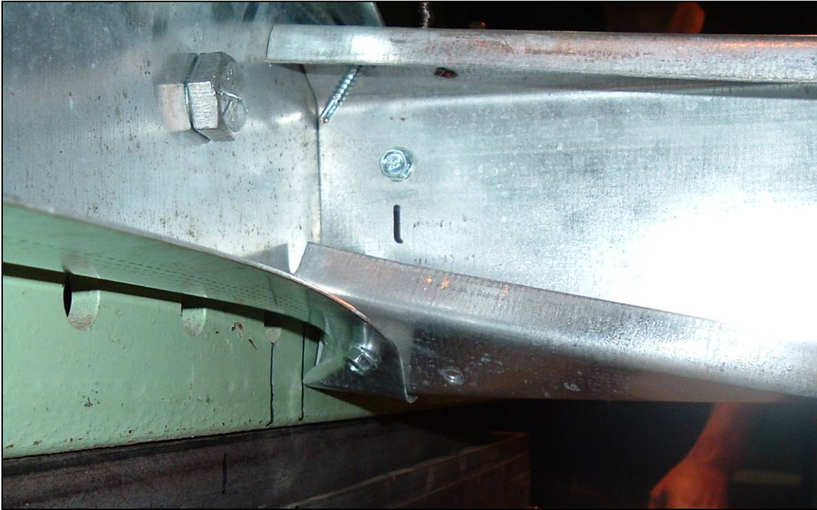
Figure 4-3: Photograph of Track Punch-Through (Specimen TS5-44-2)
