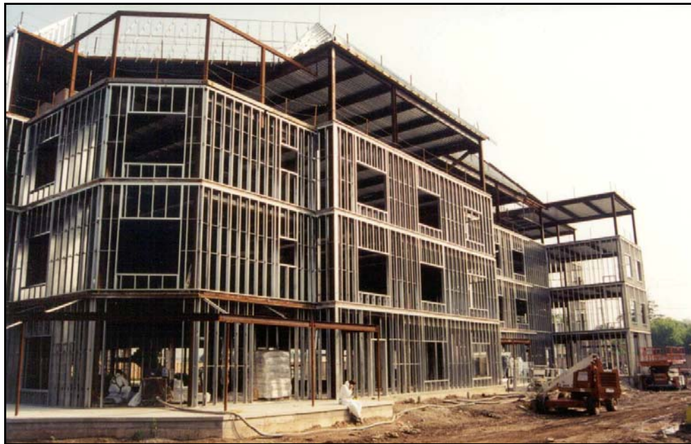
Figure 1-1: Curtain Wall Construction
