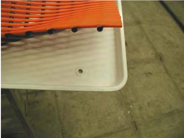
Photo 11 – Drainage for Each Rack
