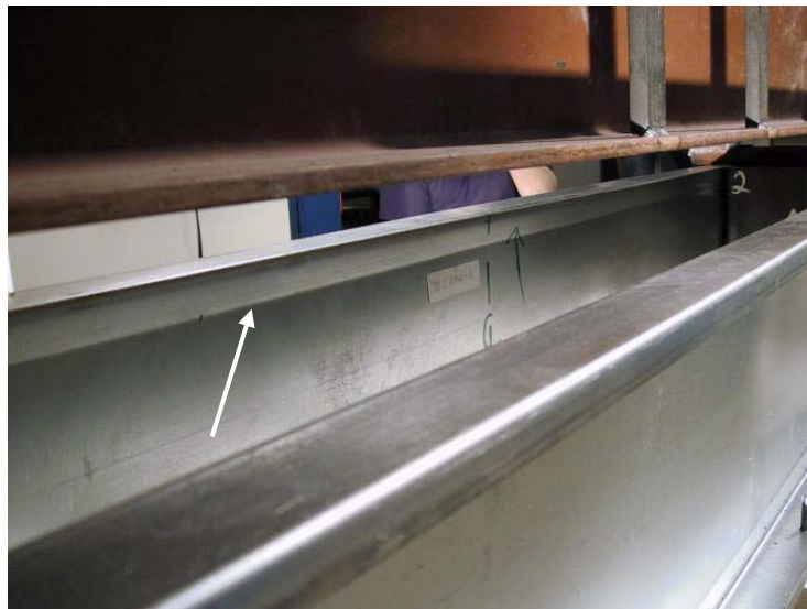
Figure 3.39 Initial damage of test D10C056-3E4W
