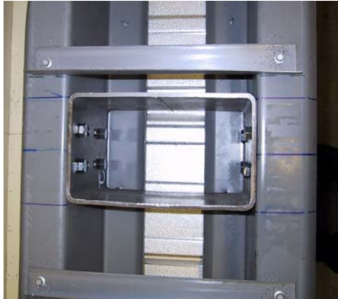
Figure 2.7 Hot-rolled tube section and angle screwed to tension flange (view from bottom)
