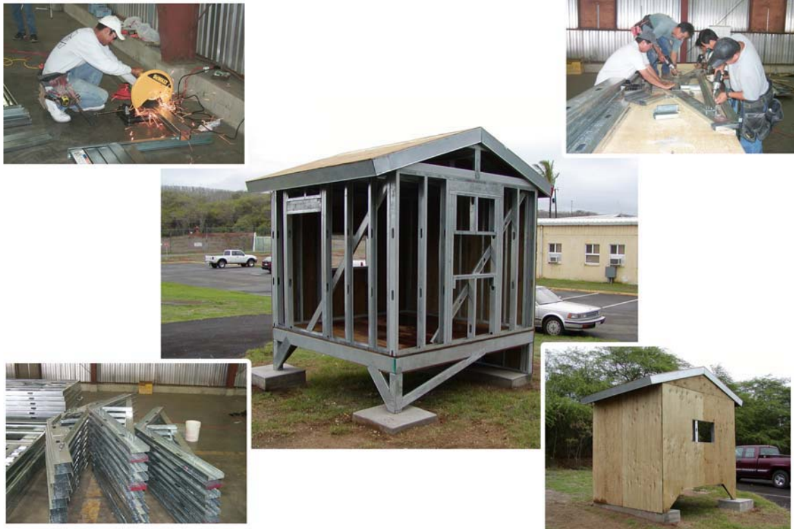
Figure 2.16: Field Enclosure at Various Stages of Construction
