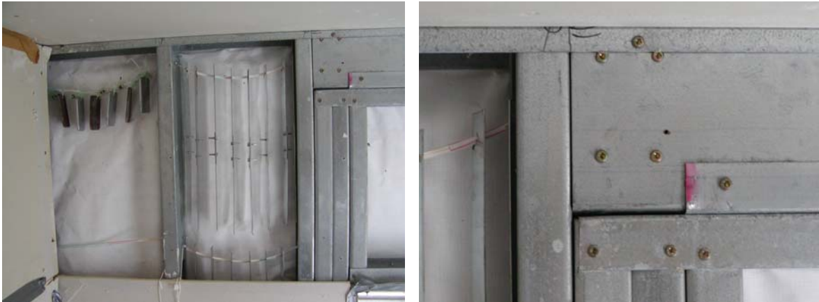
Figure 7.6: Wall framing with vapor barrier at MCBH Inland after 28 months exposure.
