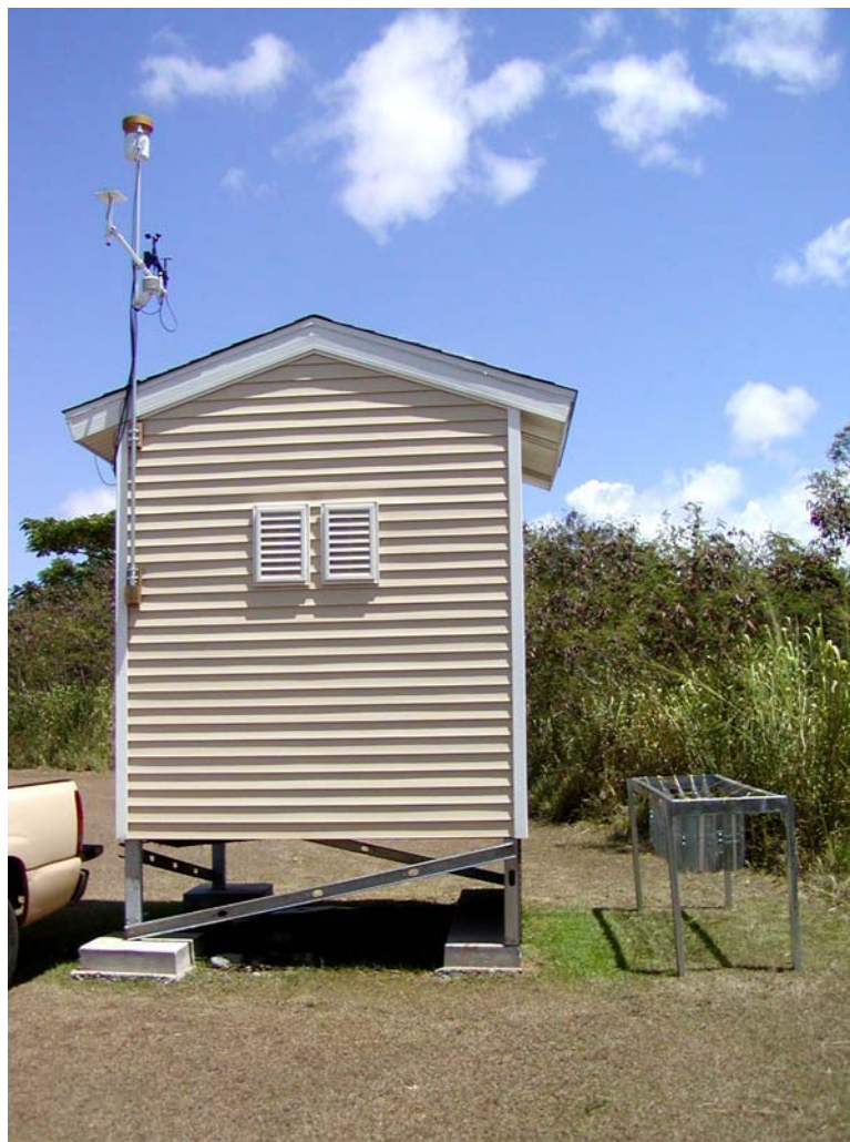
Figure 2.15: Wheeler field enclosure looking Northeast
