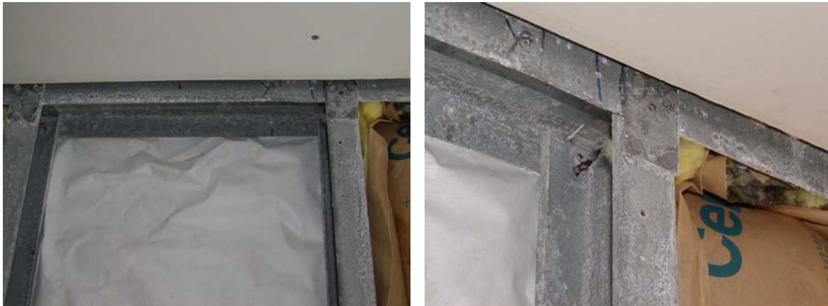
Figure 7.16: Wall framing with lap siding and vapor barrier, MCBH Coastal after 16 months.
