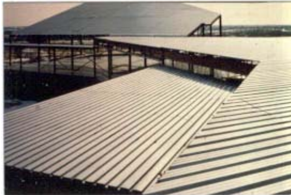
Figure 1.2-2: Cold Formed Steel Roof Decking
