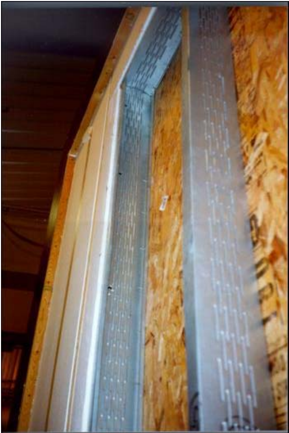
Figure 14 – Slit-Web Stud Wall Assembly
