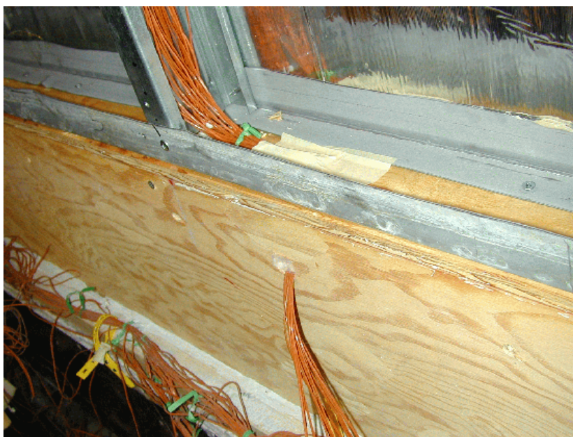
Figure 18 – Typical Split Track (Angles)
