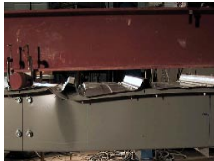
(b) Collapse of 8.5 in. Z, t=0.059 in. (nominal)
