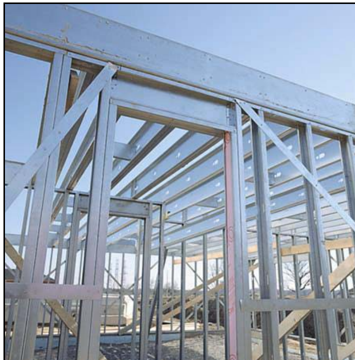
Figure 1.1.1: Photograph Showing LSF Residential Construction
