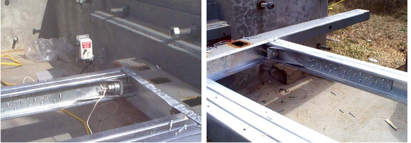
Figure 23- walls showing tie-down anchors attached to the end studs
